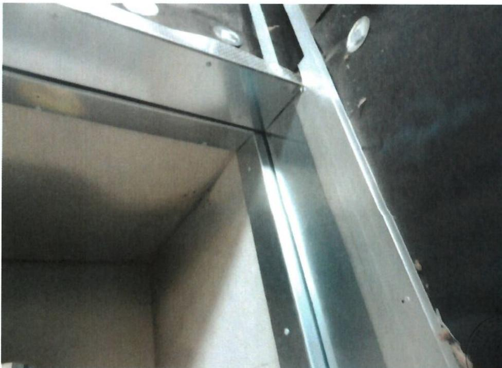
Fig. 4 (P1110012): Detail: Lintel and soffit metal facing
