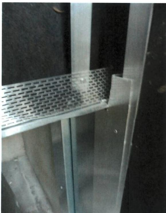
Fig. 2 (P1110007): Detail: Lintel and soffit metal facing
