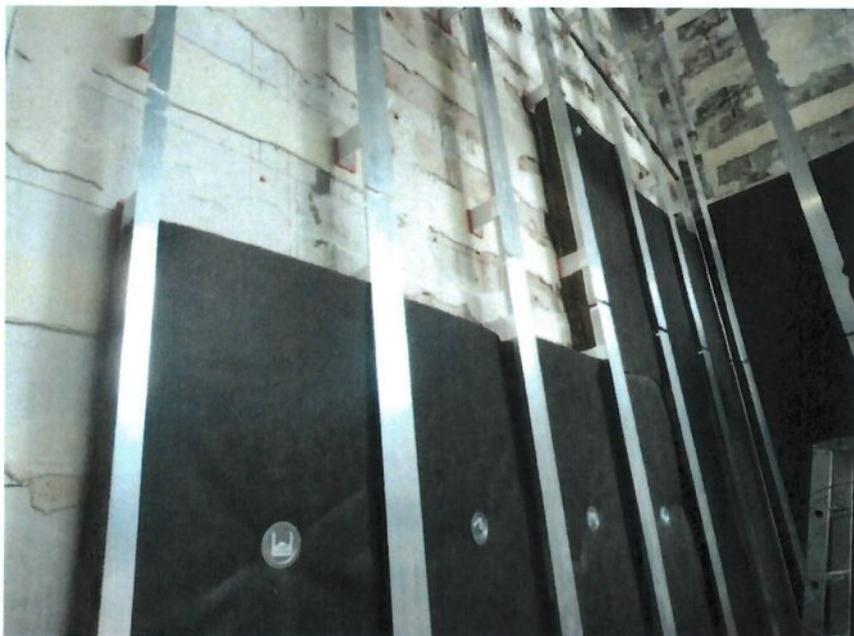
Fig. 1 (P1110001): Mounting the substructure and insulation material
