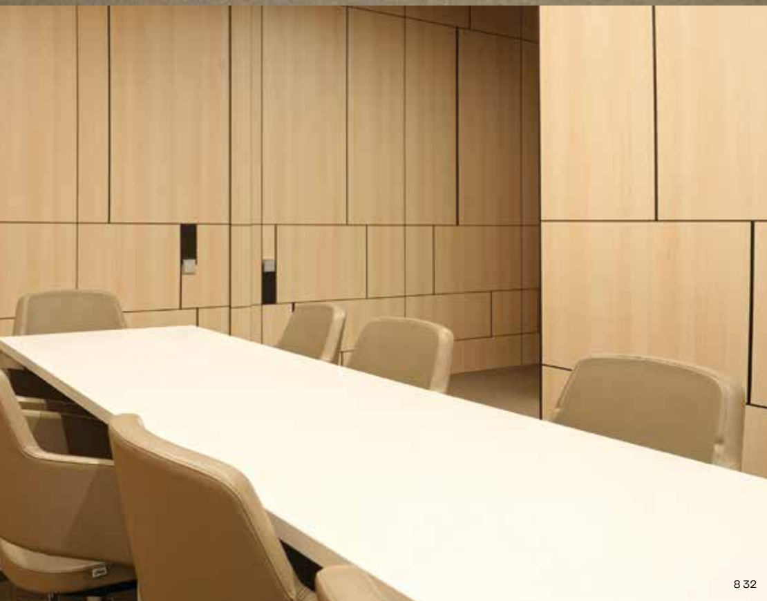
8 31 Wall cladding directly glued 8 32 Wall cladding directly glued
